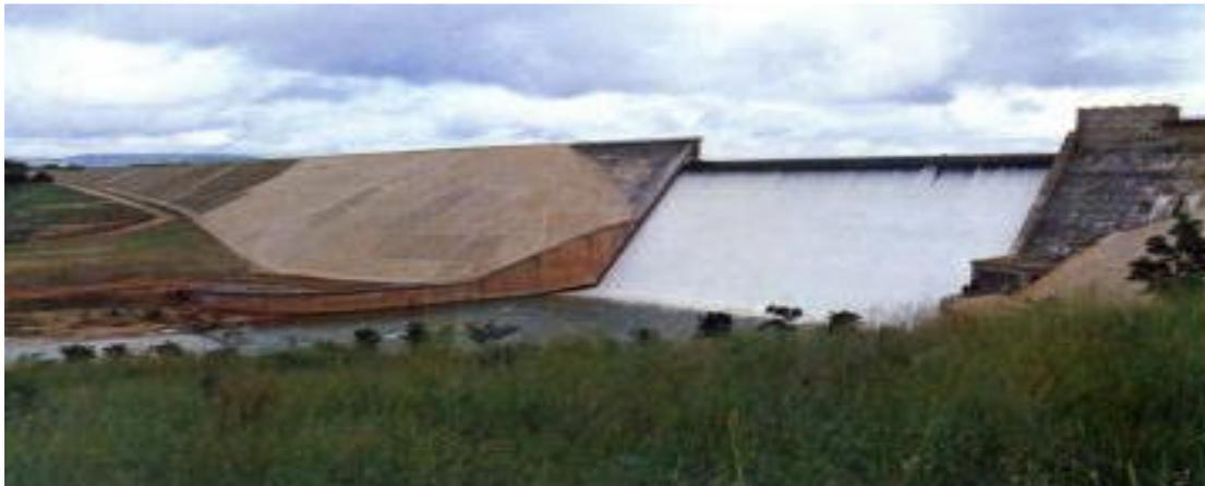
Tzaneen Dam was constructed mainly to meet the irrigation water demands along the Groot Letaba River valley. The irrigation water is released directly to the Groot Letaba River by means of a system of pipe outlets. The released water is abstracted directly from the river by pump irrigators and also diverted from the river by diversion weirs. The weirs also serve of providing reserve storage and the water is conveyed from these weirs to the irrigators by means of a bulk water supply canal.
